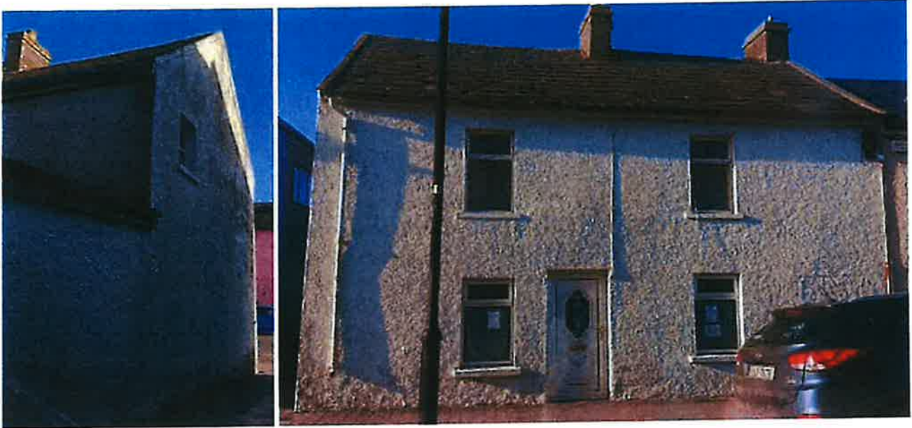
Images K & L above from 28 th March 2025, side elevation and front elevation with damaged roof, gutter, downpipe and flaking paintwork. No change in the condition of the property at Main St., Ardmore.
